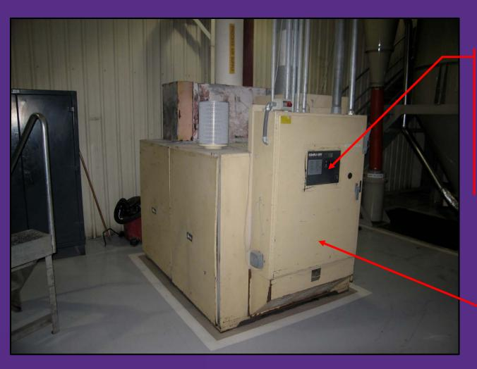
Single frequency blower produced lots of noise, vibrated floor & enclosure panels
