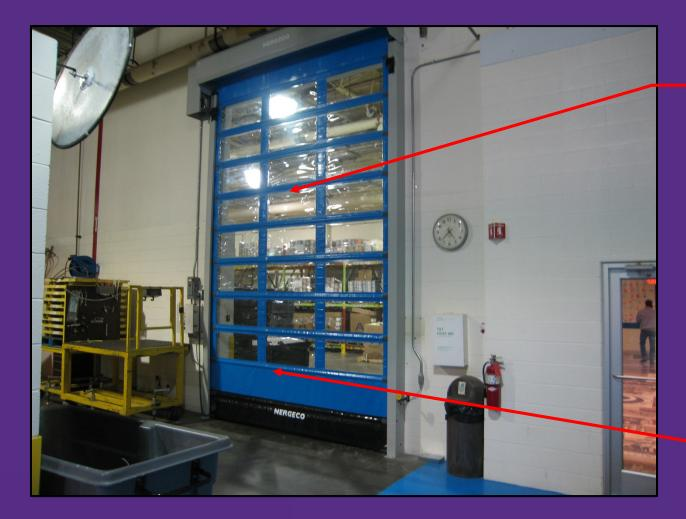
Door isolates grinder noise and HDPE dust
