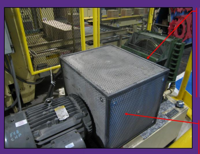
Installed suppressor to minimize hydraulic banging. Pump whine contained in sound-insulated box
